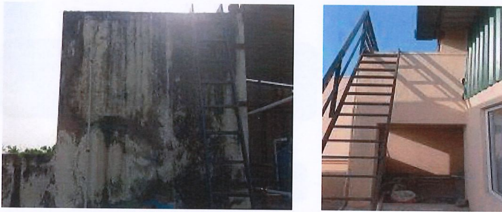
Figure 4-3: RCC overhead tanks at A-block & B-block
