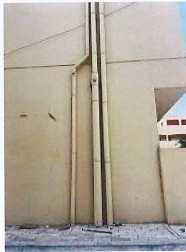
Figure 4-15: Pipelines for rain water
