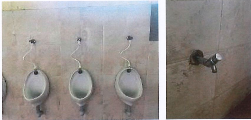
Figure 4-13: Push type tap for urinals
