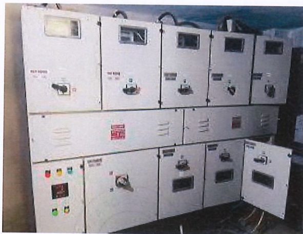
Figure 5-2: Main distribution panel
