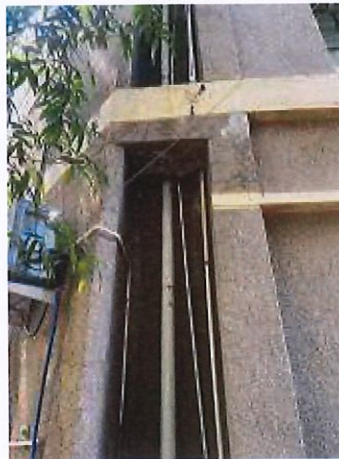
Figure 4-11: Waste water pipeline
